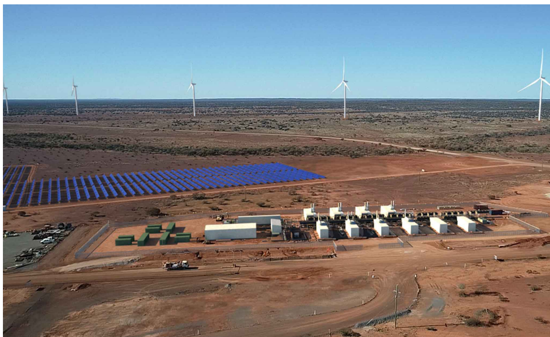
Figure 3.8 Wind turbines, solar farm and batteries at EDL's Agnew Hybrid Renewable Microgrid site
