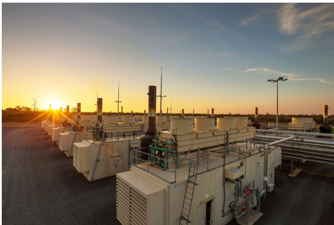
Figure 3.9 Example of power generation from coal mine methane at EDL's Moranbah North site
