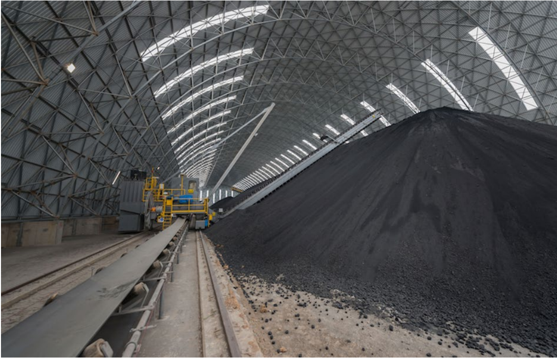
Figure 3.7 Example of enclosure for coal stockpiles
