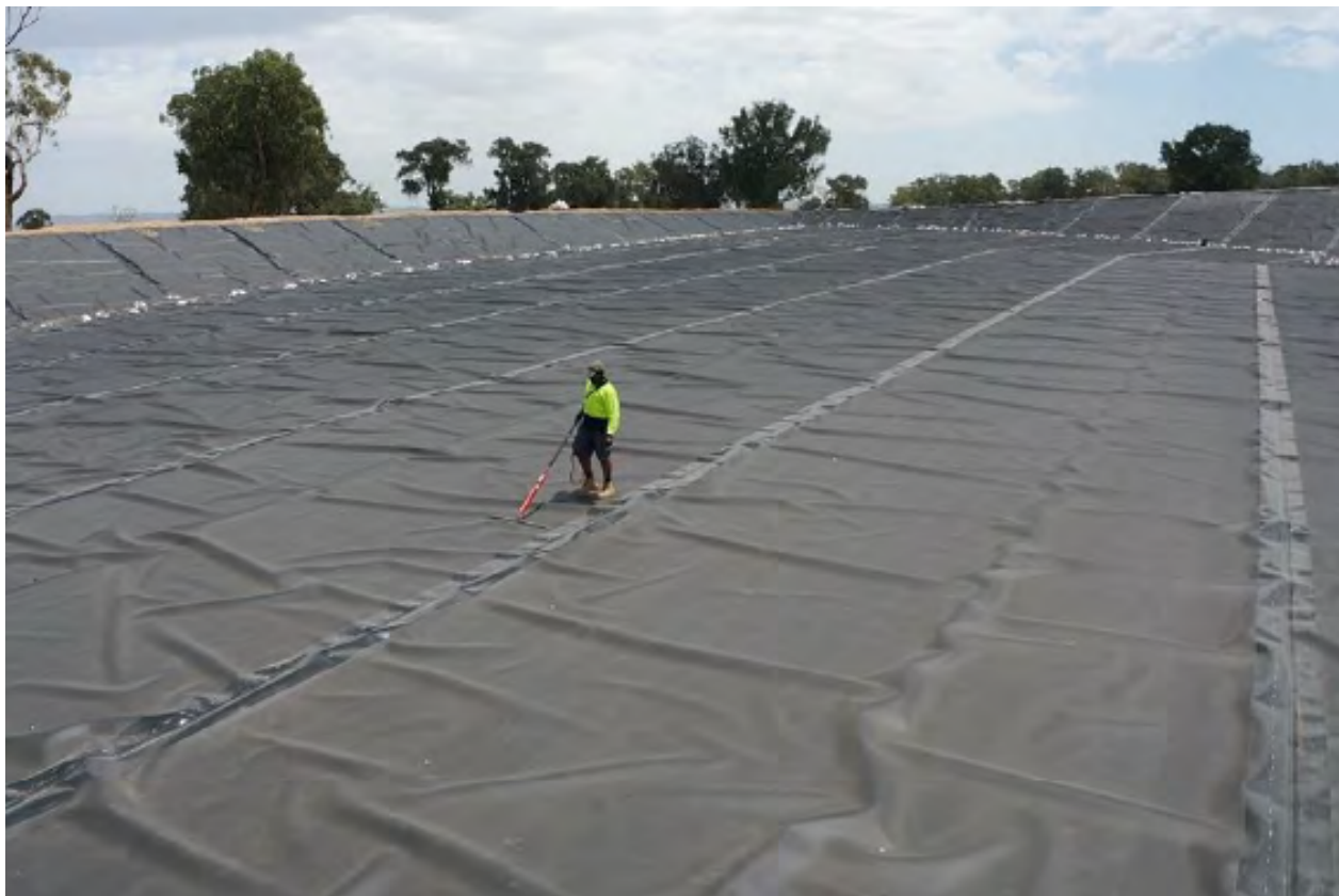
Figure 20 Leak detection following HDPE liner installation
