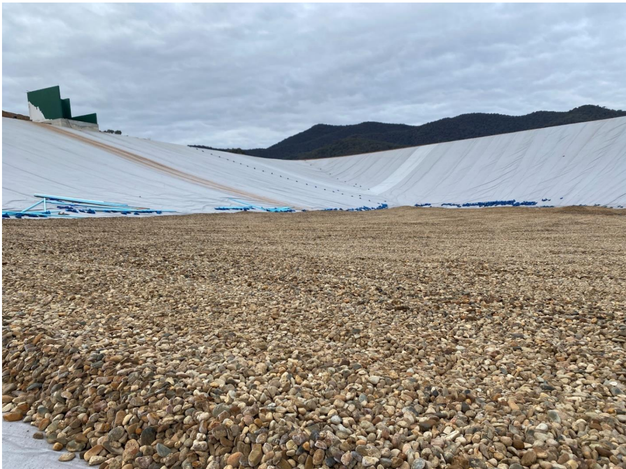
Figure 9 Protective cushion geotextile (background) and gravel drainage layer (foreground)
