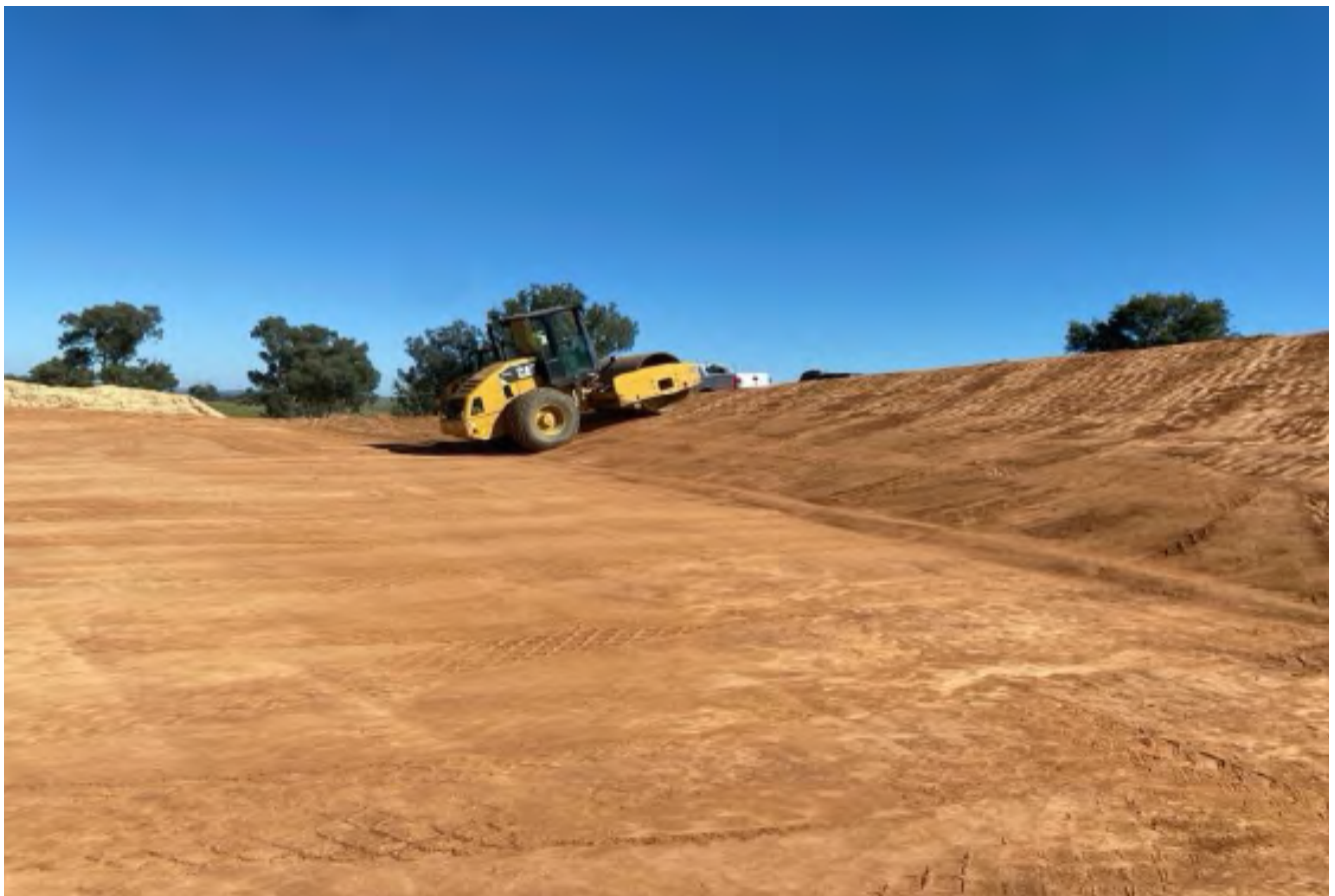
Figure 3 Compaction and smoothing of the subgrade prior to liner installation
