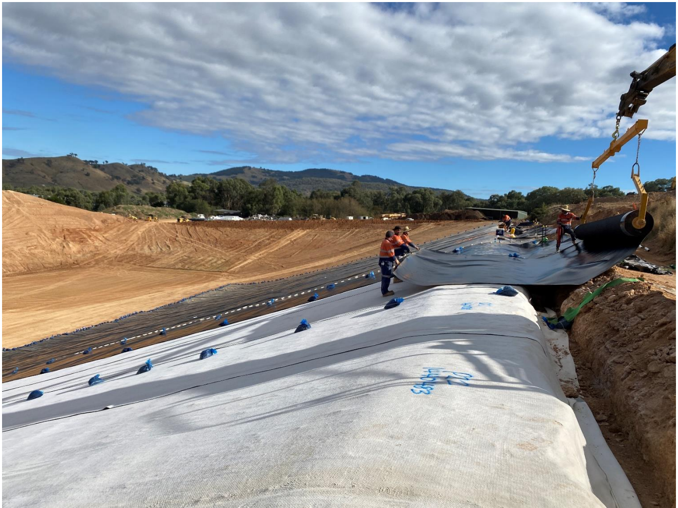
Figure 5 HDPE liner being installed over a geocomposite clay liner on the side wall with an anchor trench
