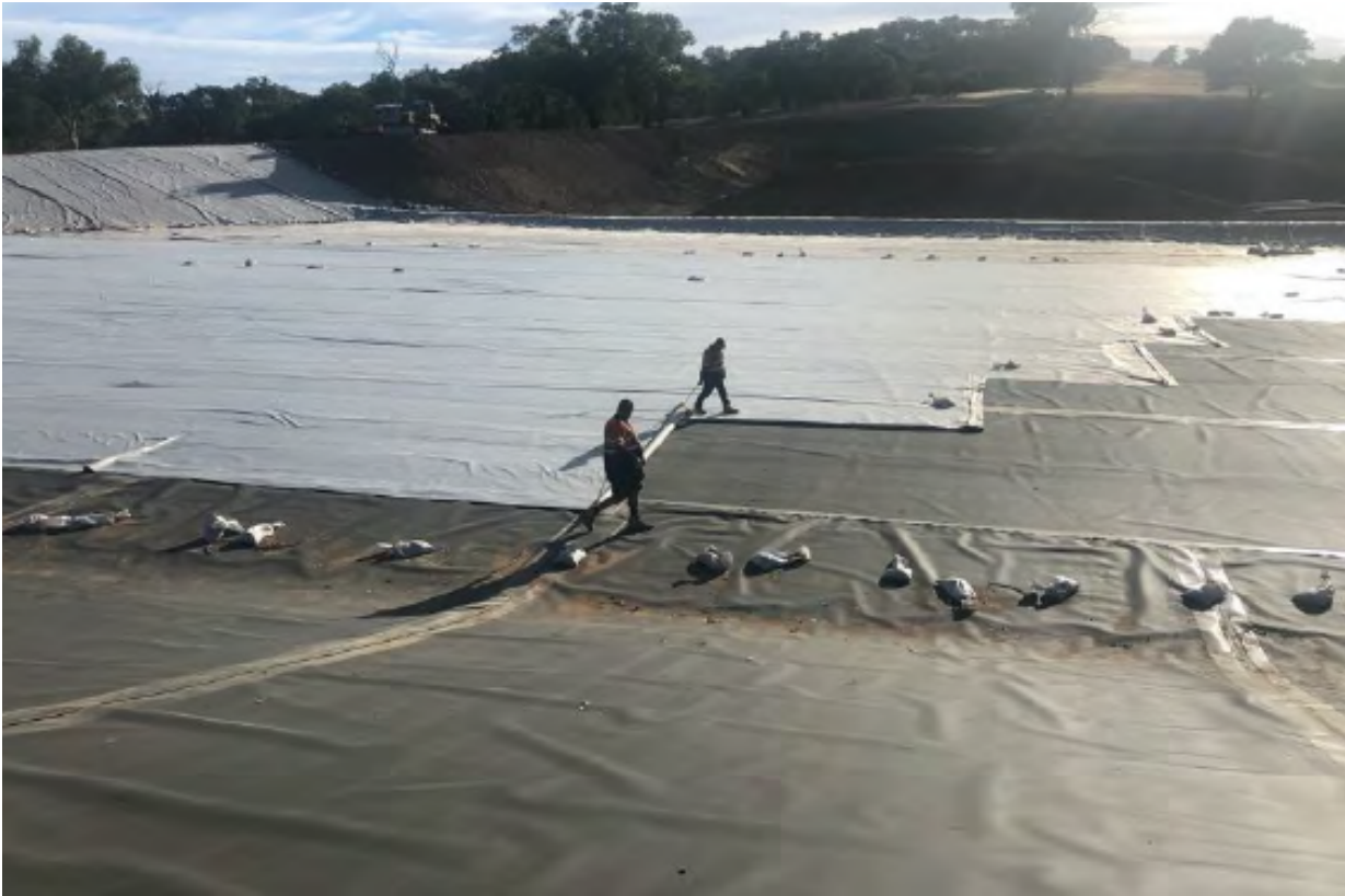
Figure 10 Applying protection geotextile to a HDPE liner
