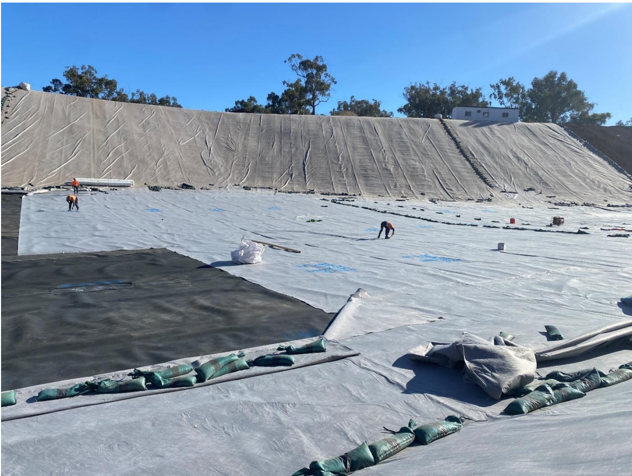
Figure 11 Applying protection geotextile to a HDPE liner
