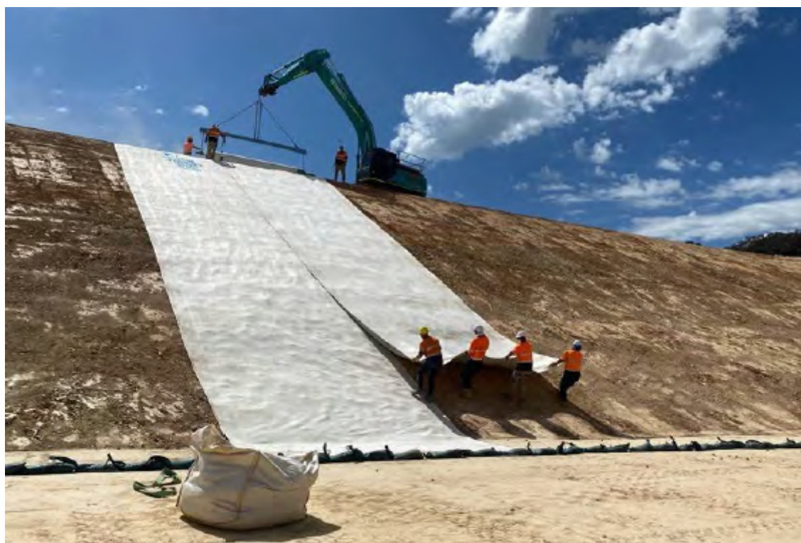
Figure 6 Installation of a geosynthetic clay liner over the sidewall
