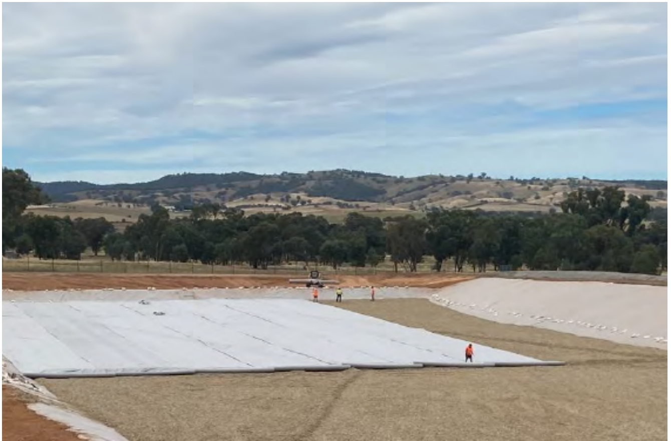
Figure 12 Applying geotextile separation layer over the gravel to minimise fines entering the leachate drainage system
