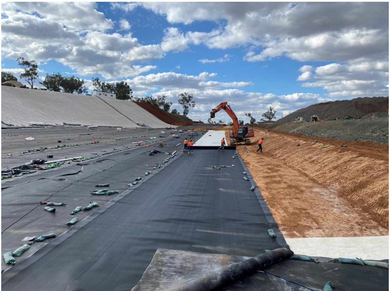
Figure 4 HDPE liner being installed over geosynthetic clay liner (GCL)
