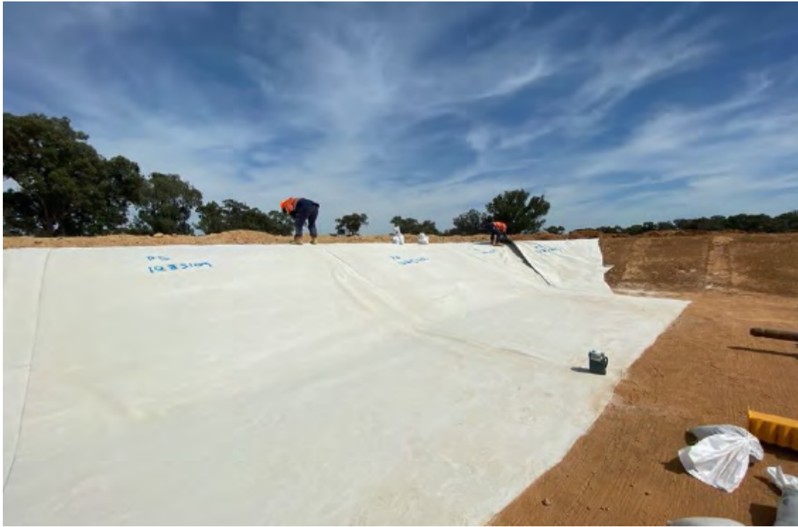
Figure 7 Installation of the geosynthetic clay liner
