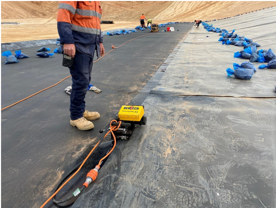
Figure 18 HDPE seam welding
