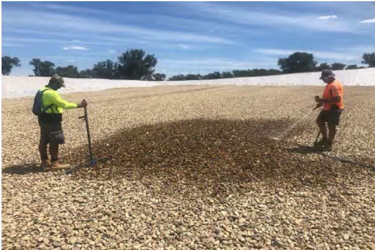
Figure 21 Leak detection of HDPE liner following installation of gravel drainage layer
